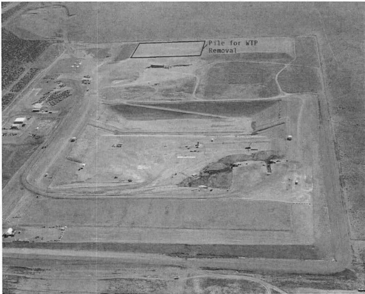
Figure 3 Aerial Photo of ERDF and Pile for WTP Removal (Looking East) - 01 May 2003
